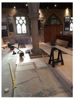
Looking towards the vestry, with the wooden flooring partly laid. At each end there is an inspection hatch for future builders, architects, wardens (!) to look underneath the floor.
