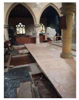
The wooden flooring is virtually complete and awaiting the oak edging. The stone flooring to the left will be a level stone surface from the vestry door to the choir stalls. The cracked monument in the floor by the vestry door will be repaired and relayed.
