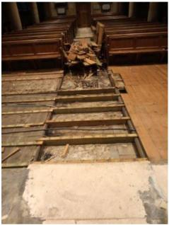
The timber flooring had been installed in the 1960.s and was of very poor quality, and after removal it was evident that the workmanship was not brilliant. The joists were supported on piles of bricks without any mortar, and worryingly the joist under the left hand front row pew had rotted through.
